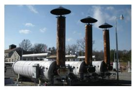
Example water bath line heater installation
